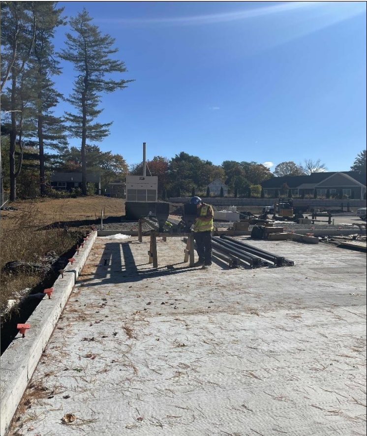
Light Poles Assembly
