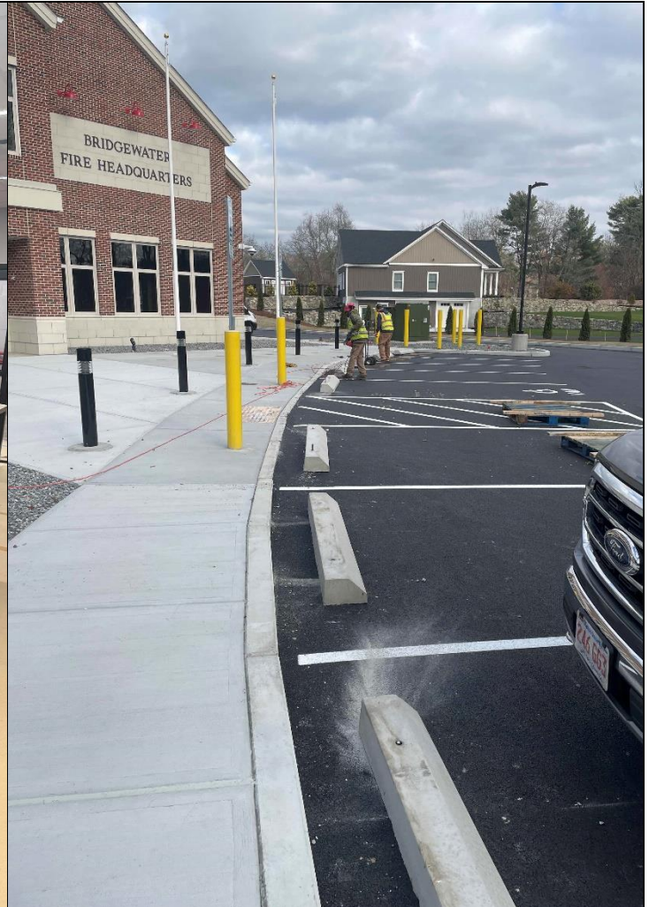
Wheel stops installed in front of the main entrance
