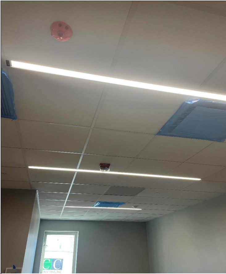
ACT Installation in Fire Prevention Room 115
