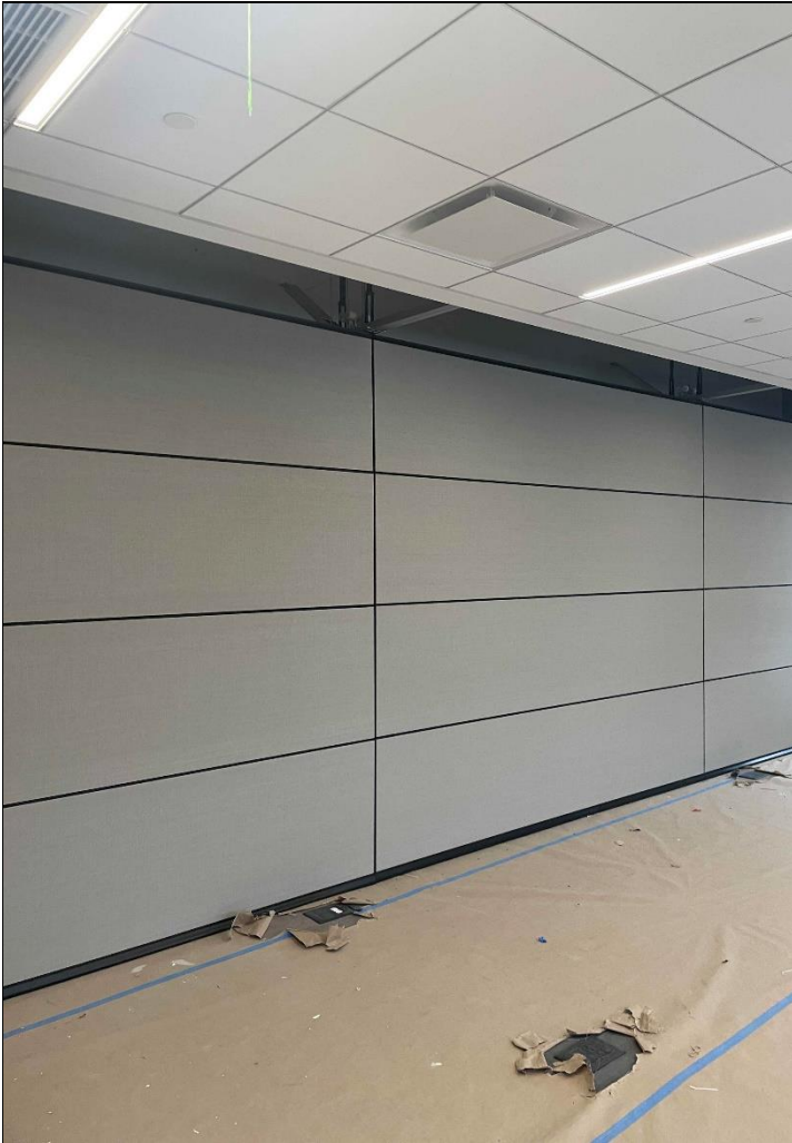
Folding partition wall installation - progress
