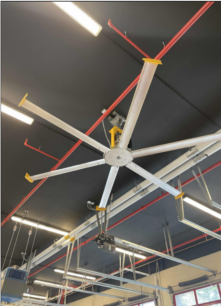
Fan Installation – Apparatus Bay
