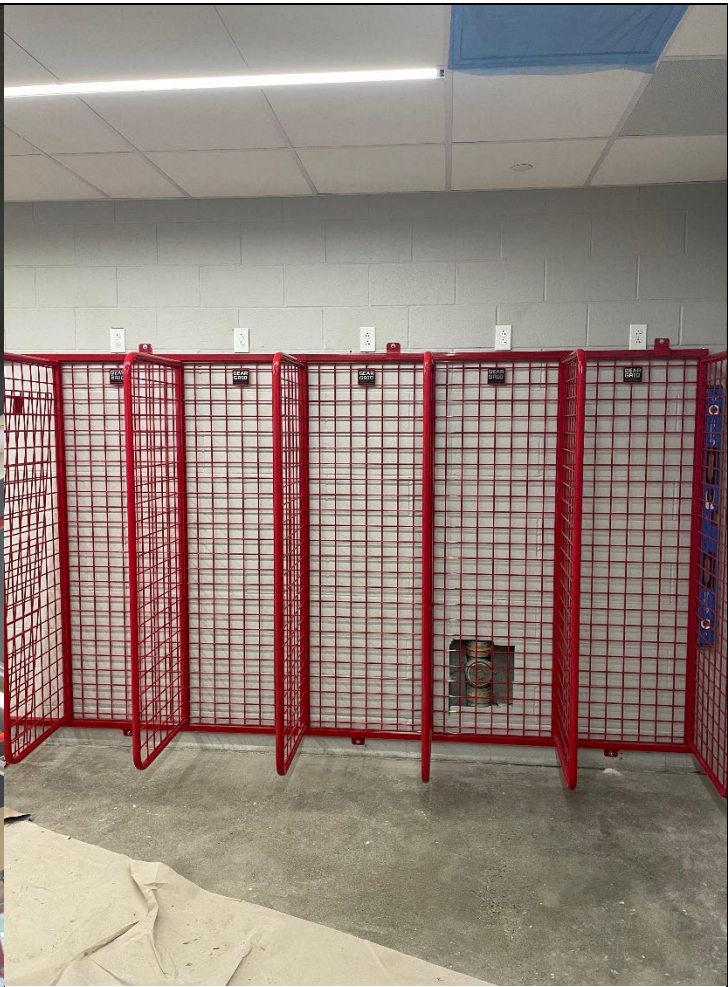
Gear grid Turnouts Installed
