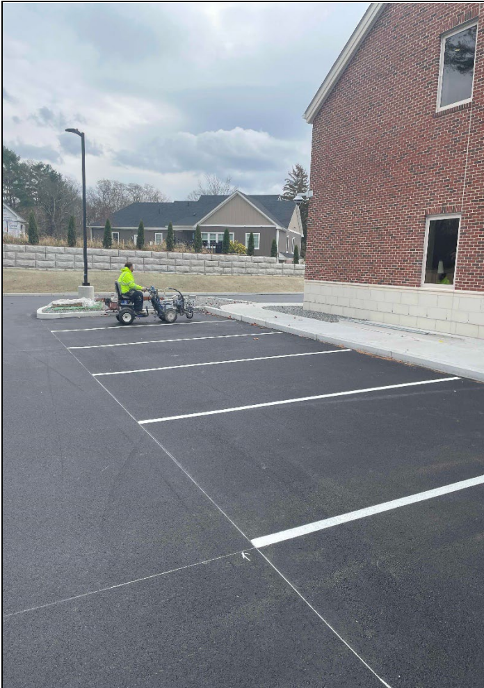
Pavement Line Striping
