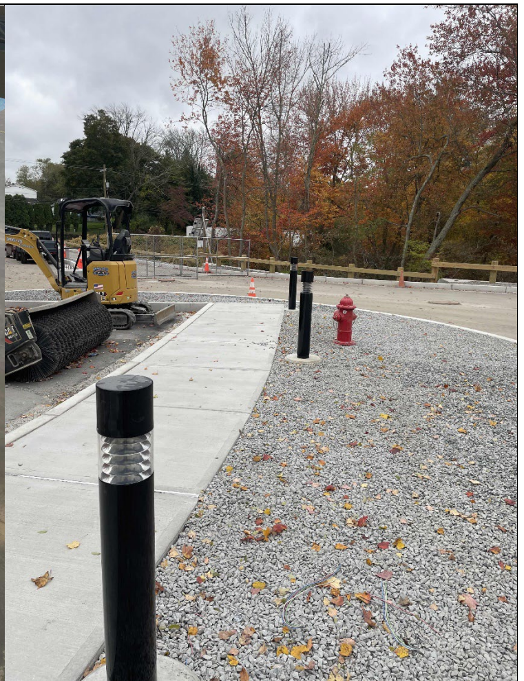
Bollard Lights Installation
