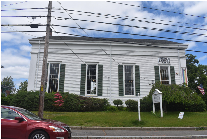
Direct view from across School St., facing north
