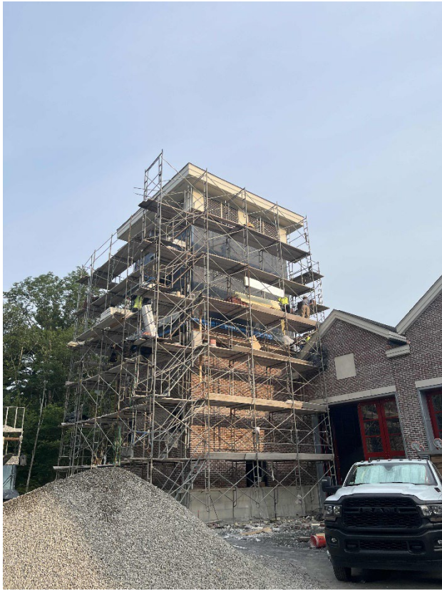
Installing rigid insulation and laying brick veneer on the Southeast elevations of the Training Tower.
