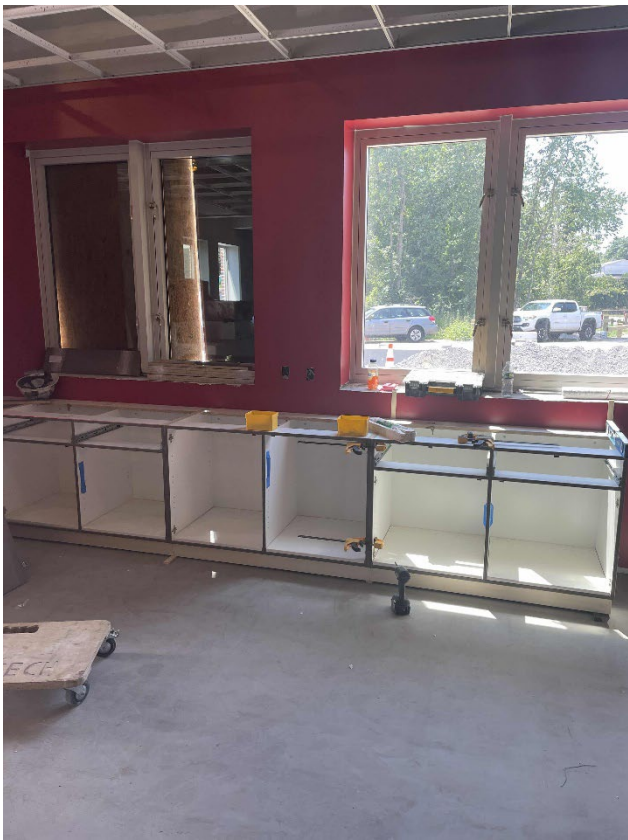
Millwork being installed in EOC/Training/Classroom 106.
