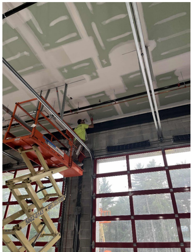
Taping Apparatus Bay ceiling.
