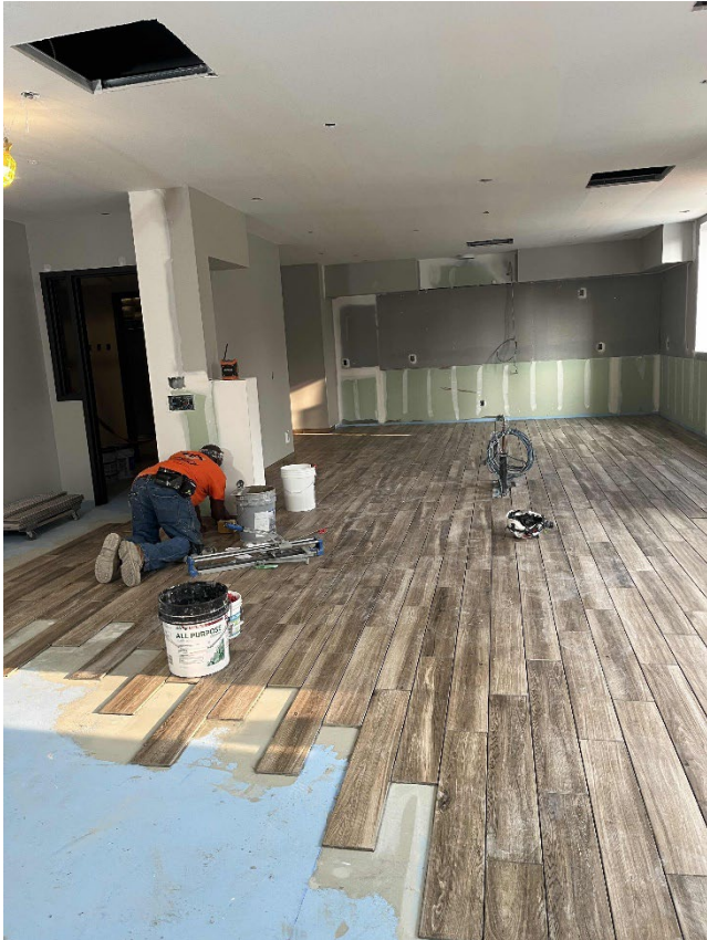
Setting floor tile in Day Room.
