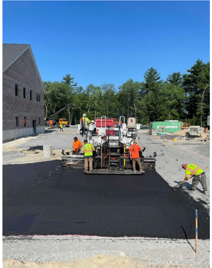
Placing the asphalt binder course
