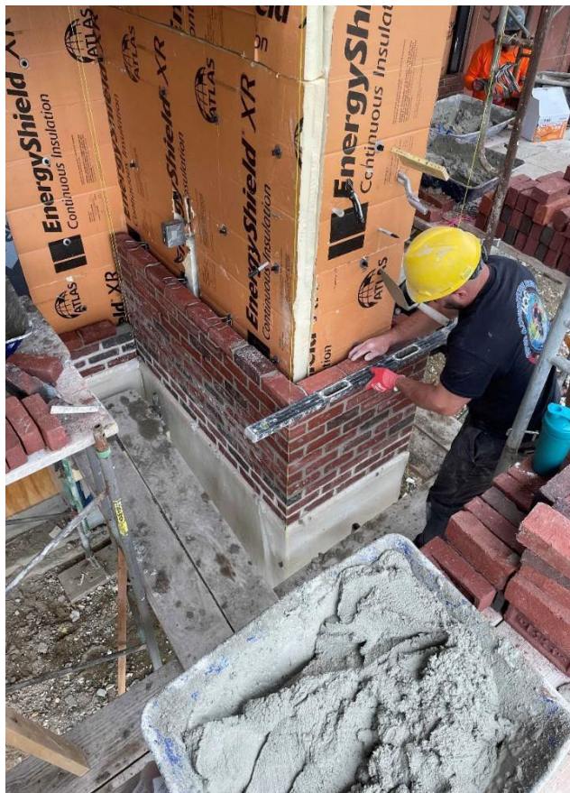
Brick façade at the main entrance
