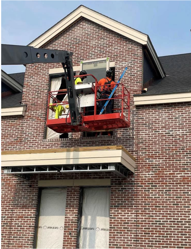
Installing windows on the east elevation
