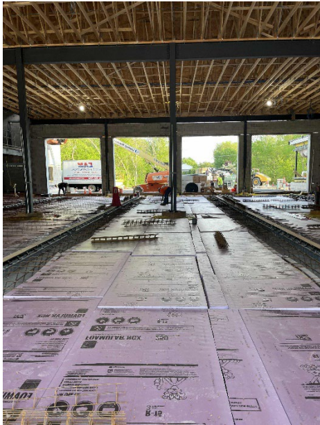
Laying Down Reinforcement in Apparatus Bay
