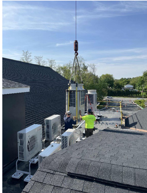
Setting RTU Condenser on Roof
