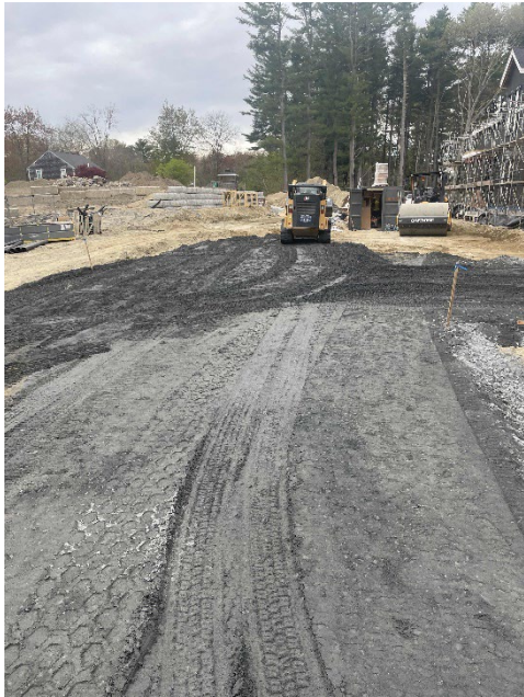
Placing Dense Grade on the East side
