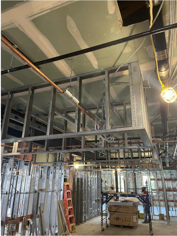
Machinical Soffit Framing
