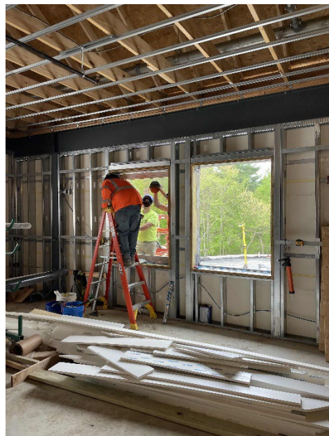
Installing Windows in Expansion Space 221
