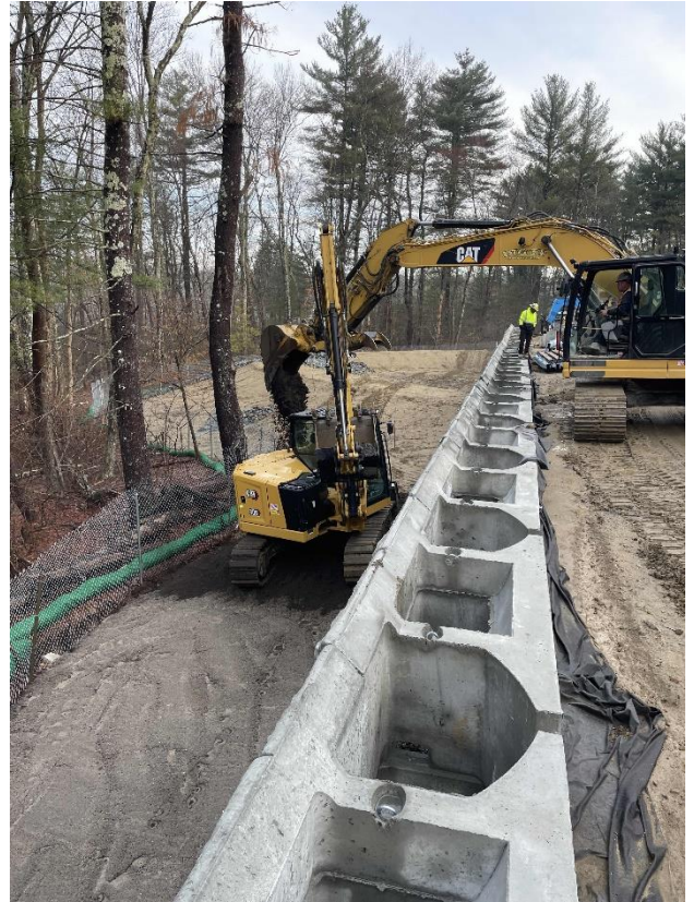
Retaining Wall Installation on the West Side
