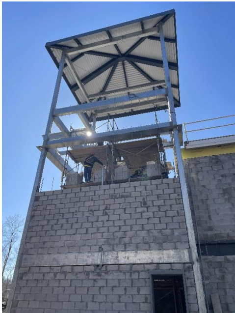
CMU Work at the Tower Stair
