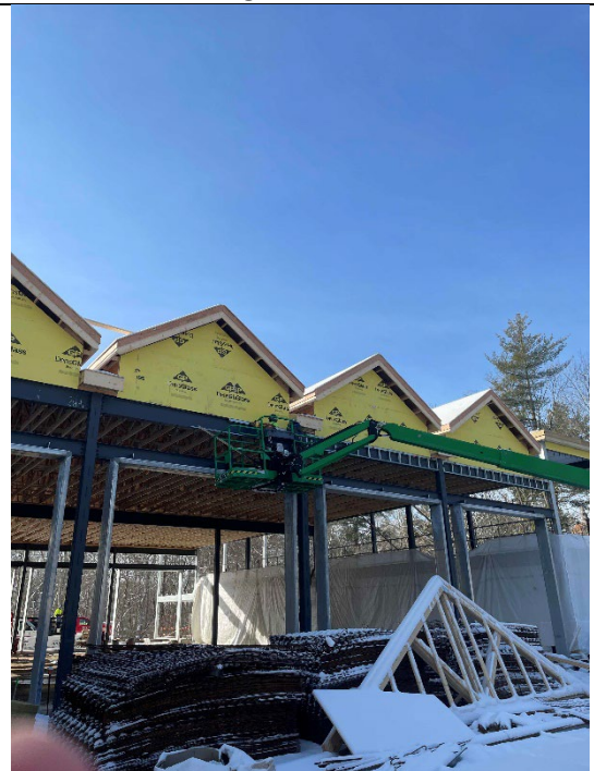
Framing and insulation above app bay door North
