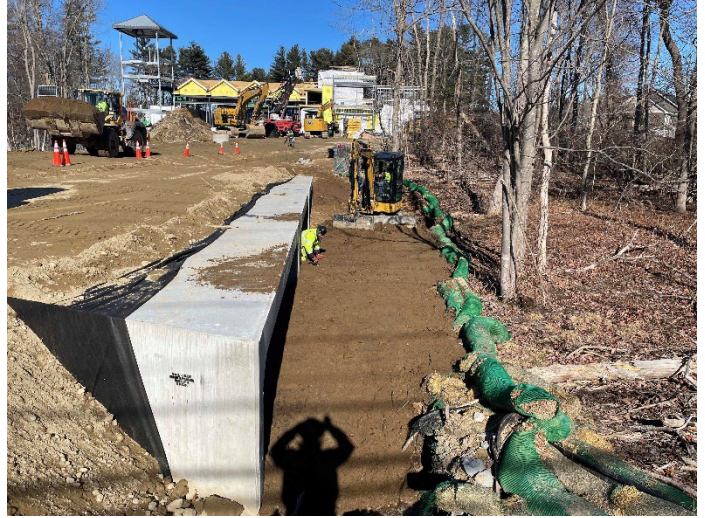
Backfilling culvert east side
