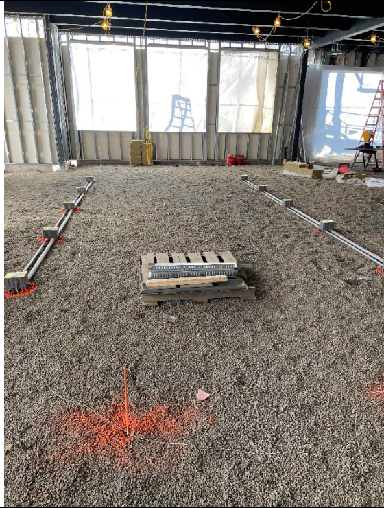
Setting floor boxes and conduits EOC/Training Classroom
