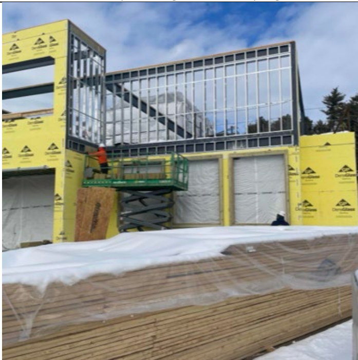
Exterior framing, sheathing and insulation progress
