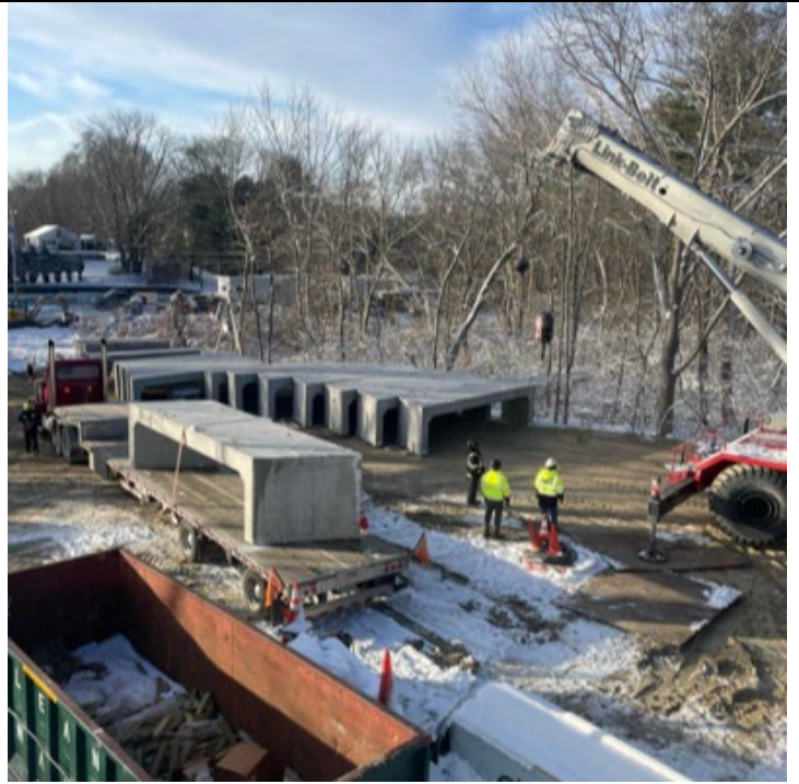
Culvert material delivery
