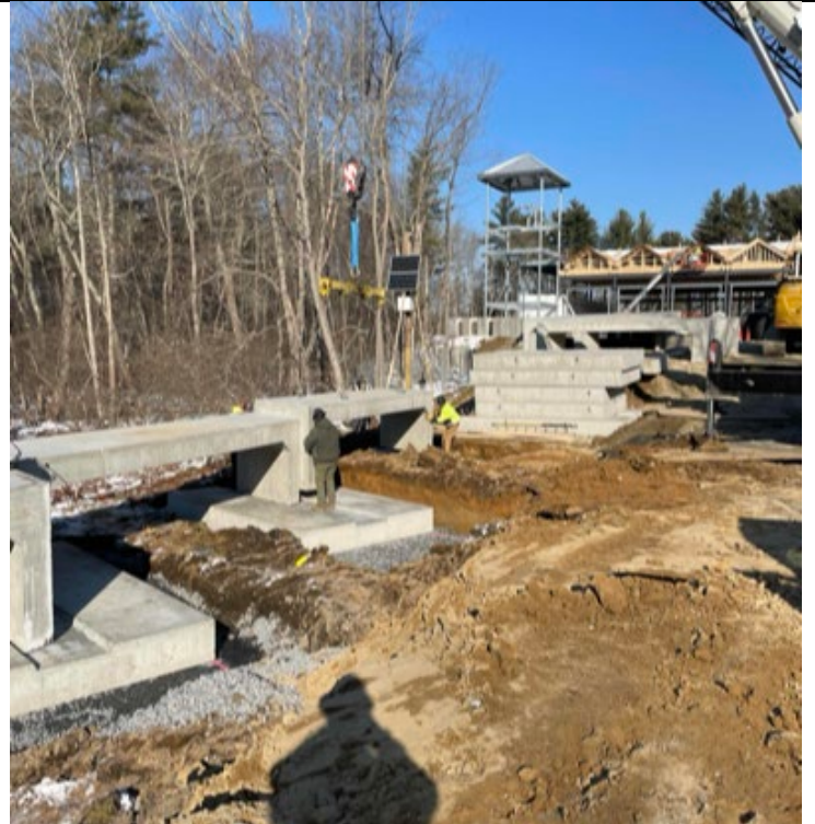
Setting culvert at west side of entrance
