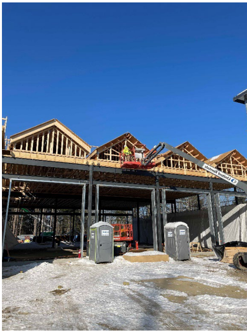
Framing the dormers on app. bay South
