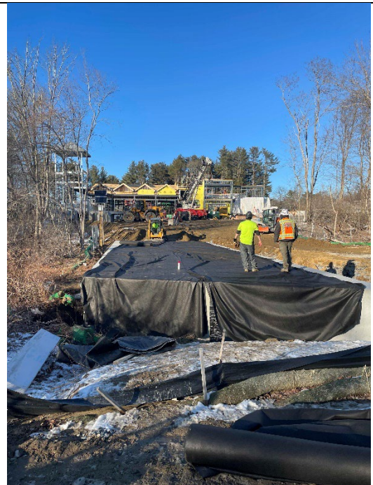
Filter fabric placed over culvert prior to backfilling
