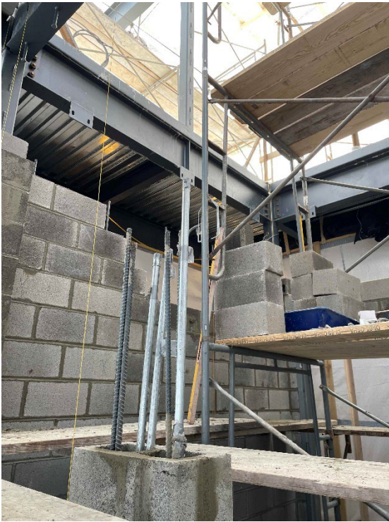
CMU Block install Stair A
