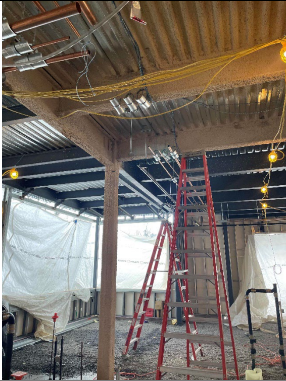
Overhead plumbing installation progress
