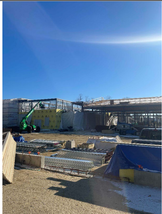
Ext. framing and app bay roof progress from N elevation
