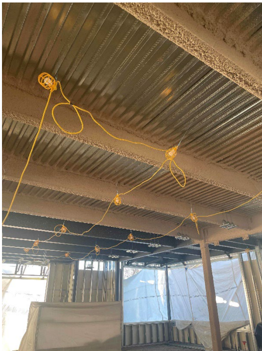
Temporary lighting installed for administration area
