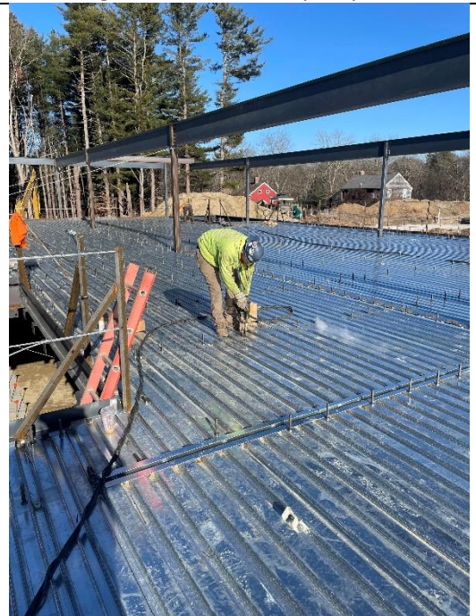
Welding shear studs for upper level slab on deck
