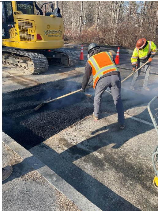
Paving the water trench on Pleasant St
