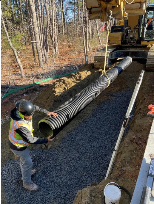
Installing drainage piping behind the outbuilding
