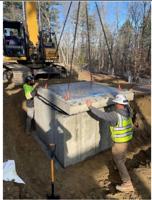
Setting the hatch for the pump chamber
