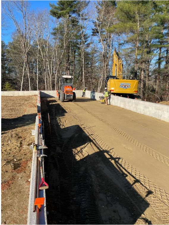
Backfilling inside the outbuilding foundation
