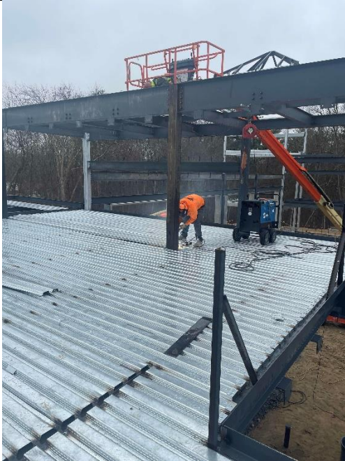
11.21.24 Metal Decking Detailing
