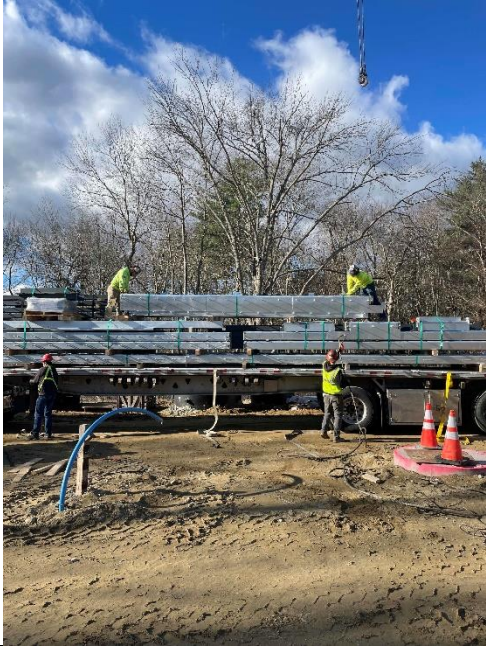
11.12.24 Galvanized Steel Delivery
