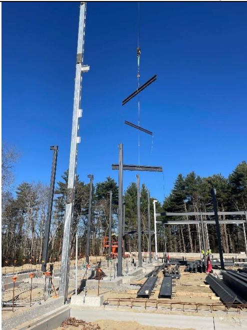
11.14.24 Sequence 3 and 4 Steel Erection
