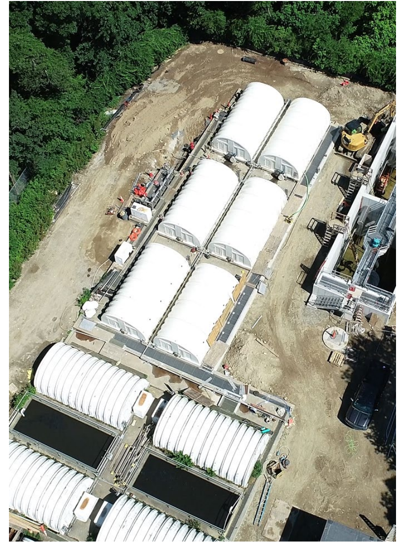
Morris Ave. WWTF Rotating Biological Contactors (Under Construction), June 2024
