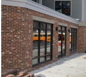
Examples of appropriate masonry walls
