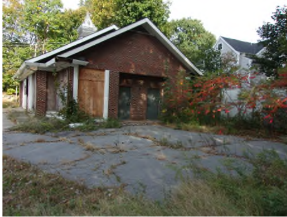
Subject Property Easterly Side View
