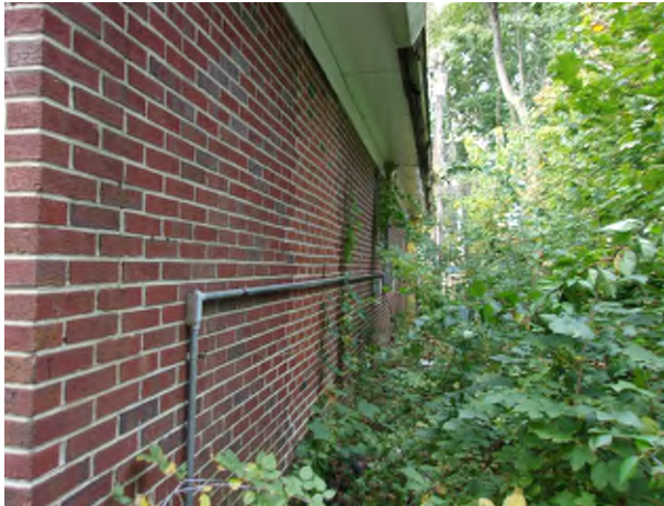
Subject Property Rear View
