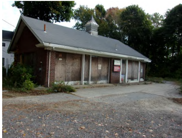
Subject Property Front / Westerly Side View
