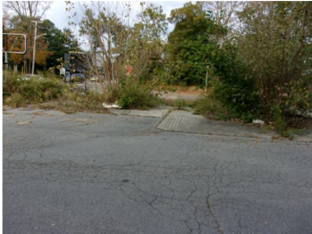
Subject Property Front Parking Area View
