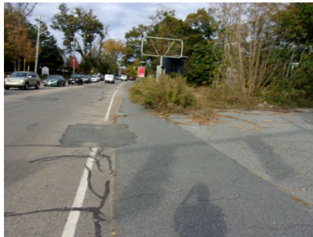
Subject Property Street Frontage View
